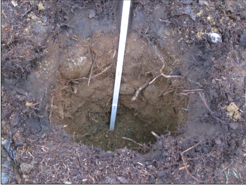
Figure 16. Typical subsurface conditions in the northwestern part of the project as seen in probe 26.
